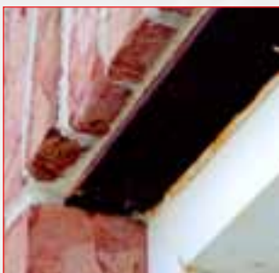
An unsightly, rusted brick angle begins staining the window frame and the bricks.
