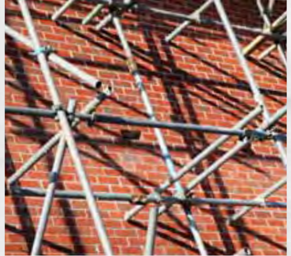
Galvanized steel makes construction forms such as scaffolding, shoring systems, and forming structures safer for workers.
