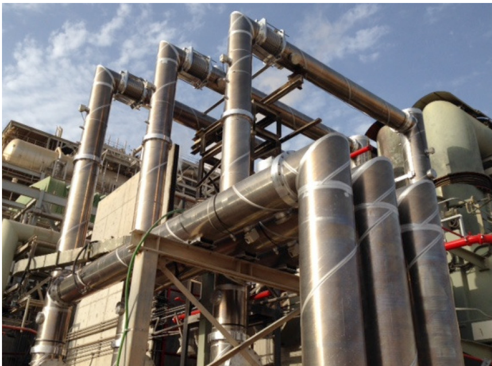
Replacement transformer with new AZZ GIL ready for energization
