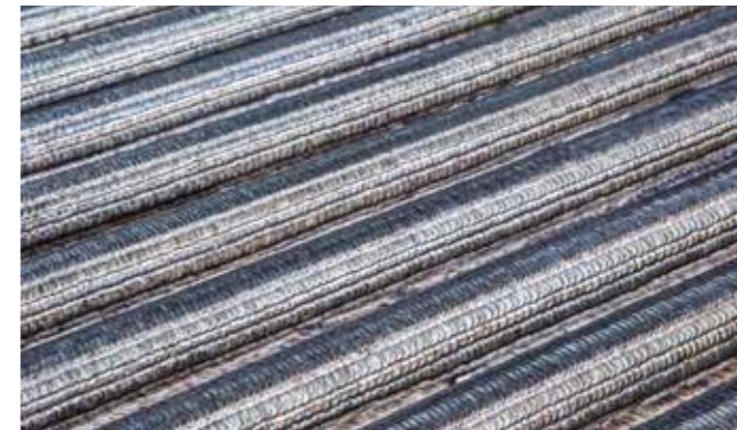
Unifuse 180 - Boiler panel life extension
