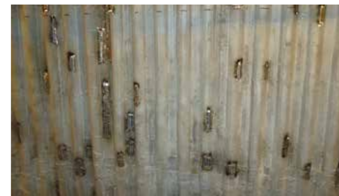
Spot repairs on an old 625 weld overlay
