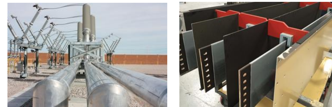
High Voltage Bus
