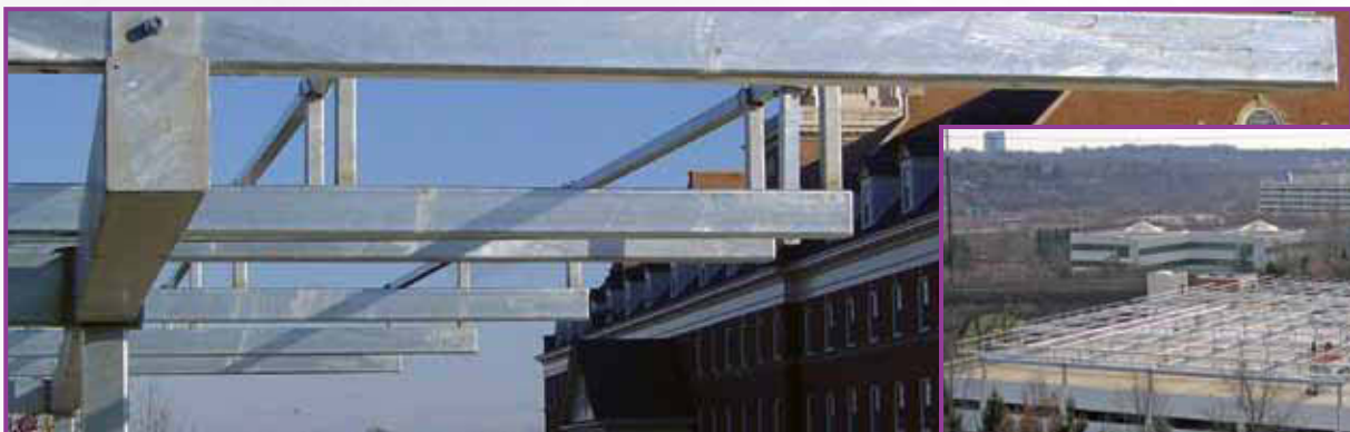
The solar roof panel system above the Johnson and Johnson building is hot-dip galvanized to withstand New England's harsh weather conditions.
