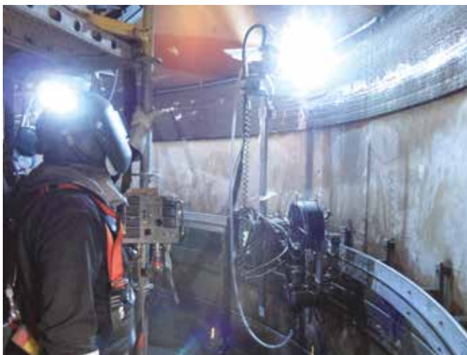
Workforce is fully equipped with necessary safety materials
