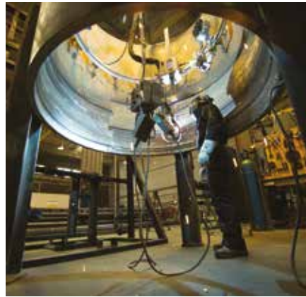
Mock-up for automatic weld overlay
