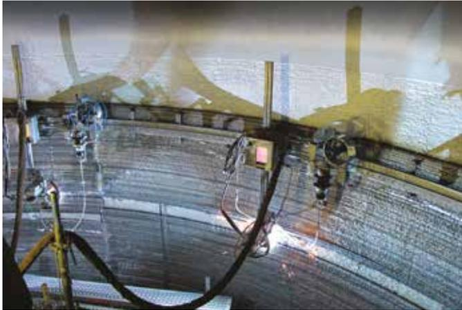
Automated weld overlay using the **Unifuse** process
