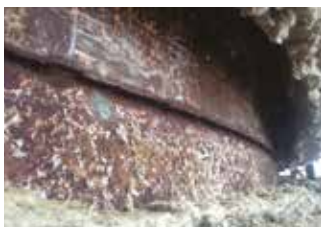
Skirt-to-shell cracking
