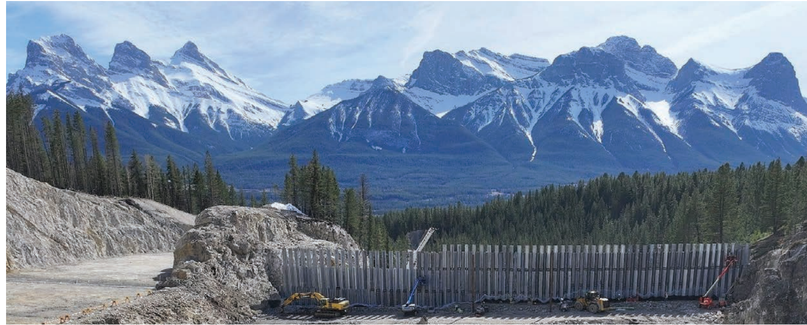
Cougar Creek Debris Flood Retention Structure in Edmonton, Canada.
